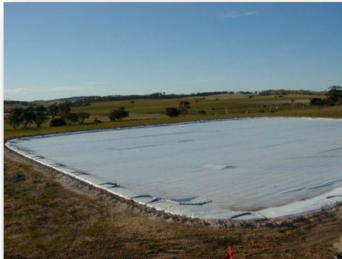
Figure 2. Evap-cap, a barrier to reduce evaporation rate.
