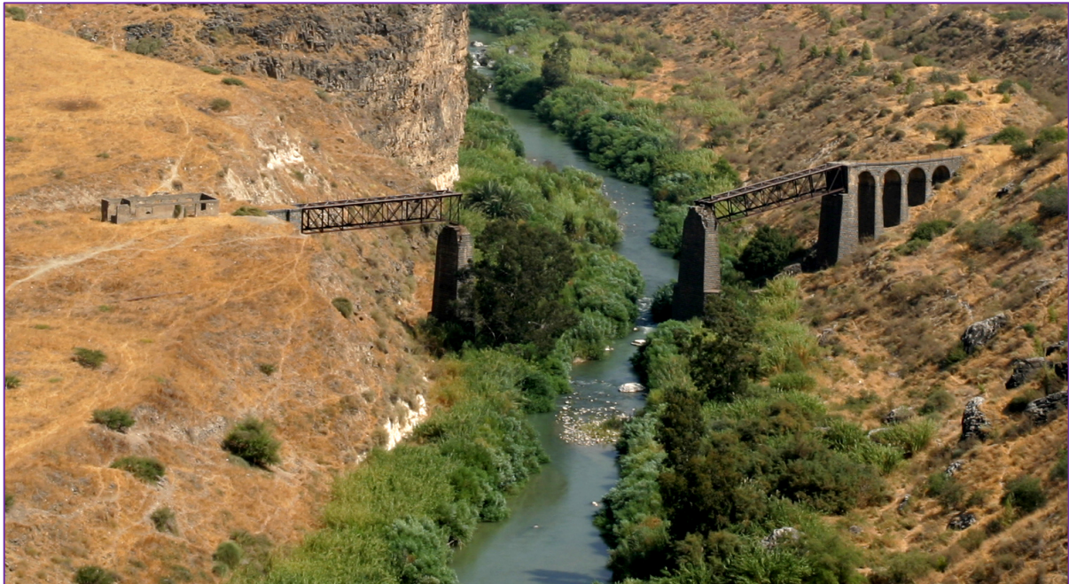
Figure 5.3 The Himmeh Bridge, bombed by the (Zionist military organisation) Haganah on 17 June 1946 as part of a plan to destroy 11 bridges linking Palestine to neighbouring Arab States. Source: Benjamin, 2004, Flickr.
