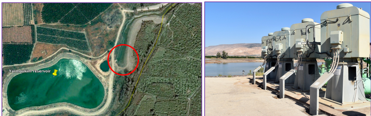
Figure 6.5 Top: The Yarmoukim Reservoir and the termination of the Yarmouk riverbed (red circle): the ‘end of the Yarmouk’. Source: Adapted from Google Earth. Bottom: The reservoir, and motors of the four pumps that abstract from the Yarmouk. Source: Authors.
